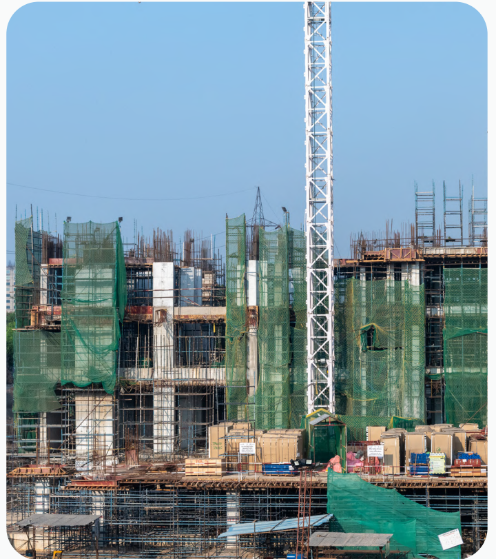
Tower D - Floor casting in progress
