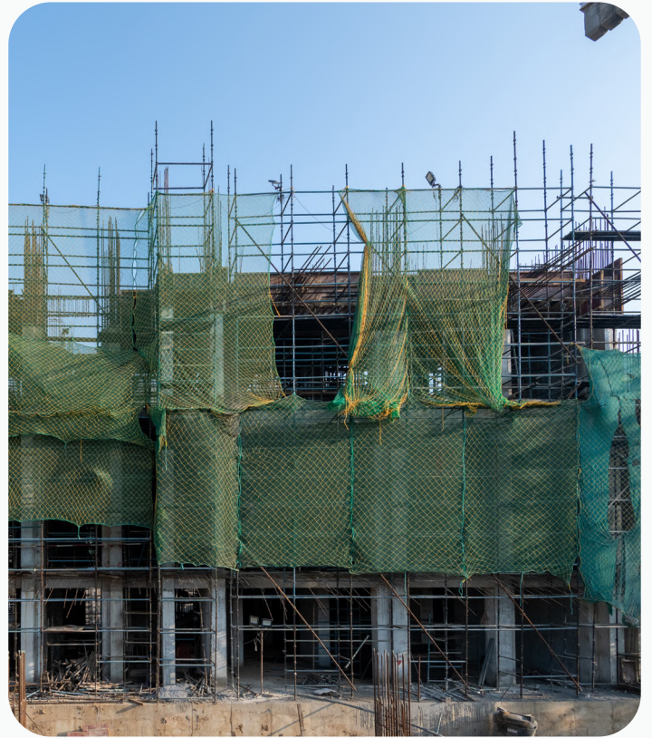
Tower B - Final basement in progress
