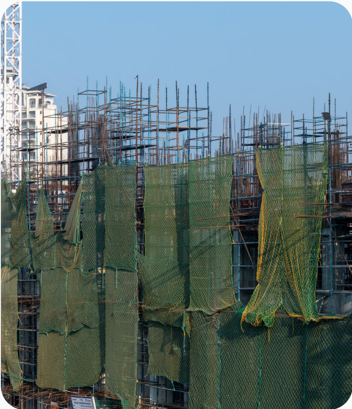
Tower C - Basement completed
