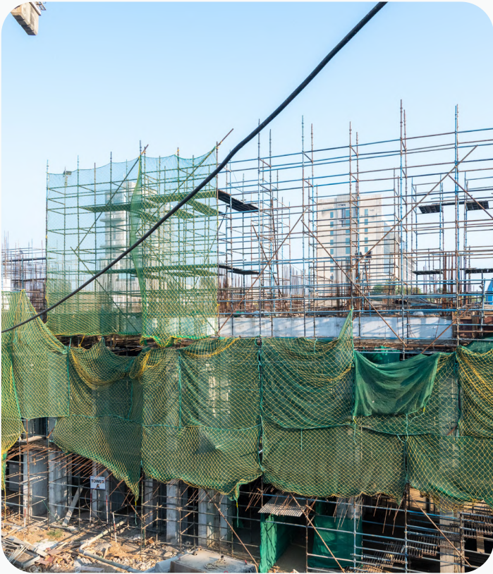
Tower A - Final basement in progress
